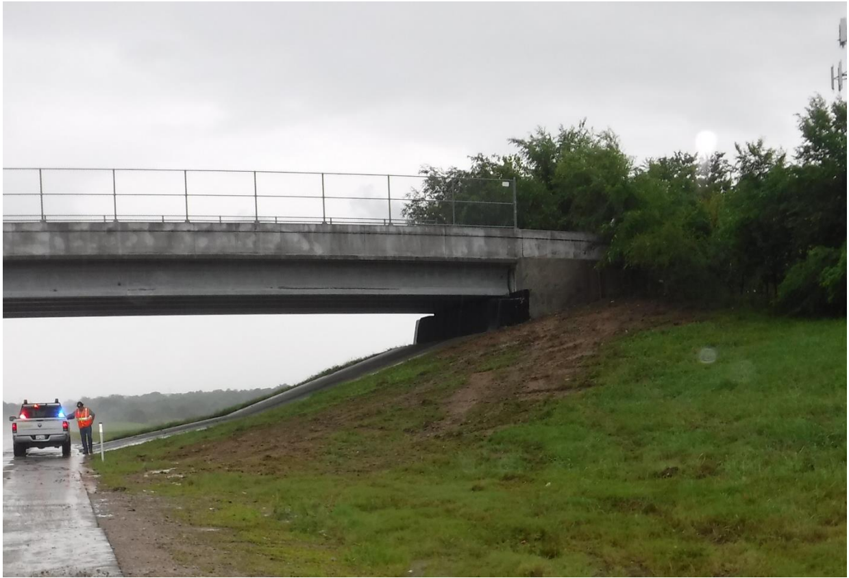
Photo 2: NW Abutment Slope
