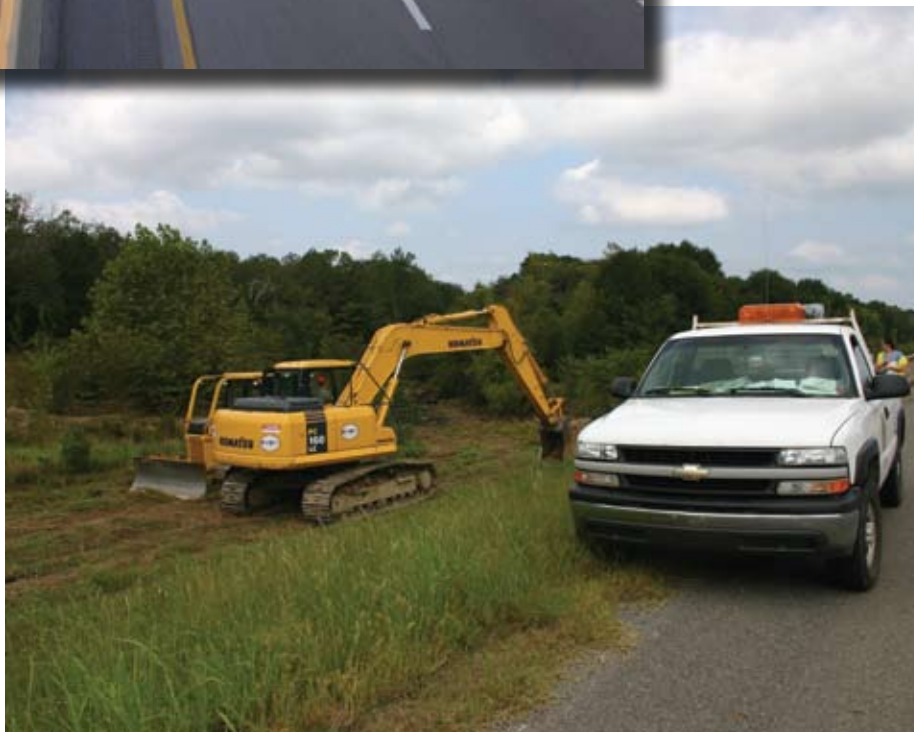
INDIAN NATION TURNPIKE - DRAINAGE WORK
