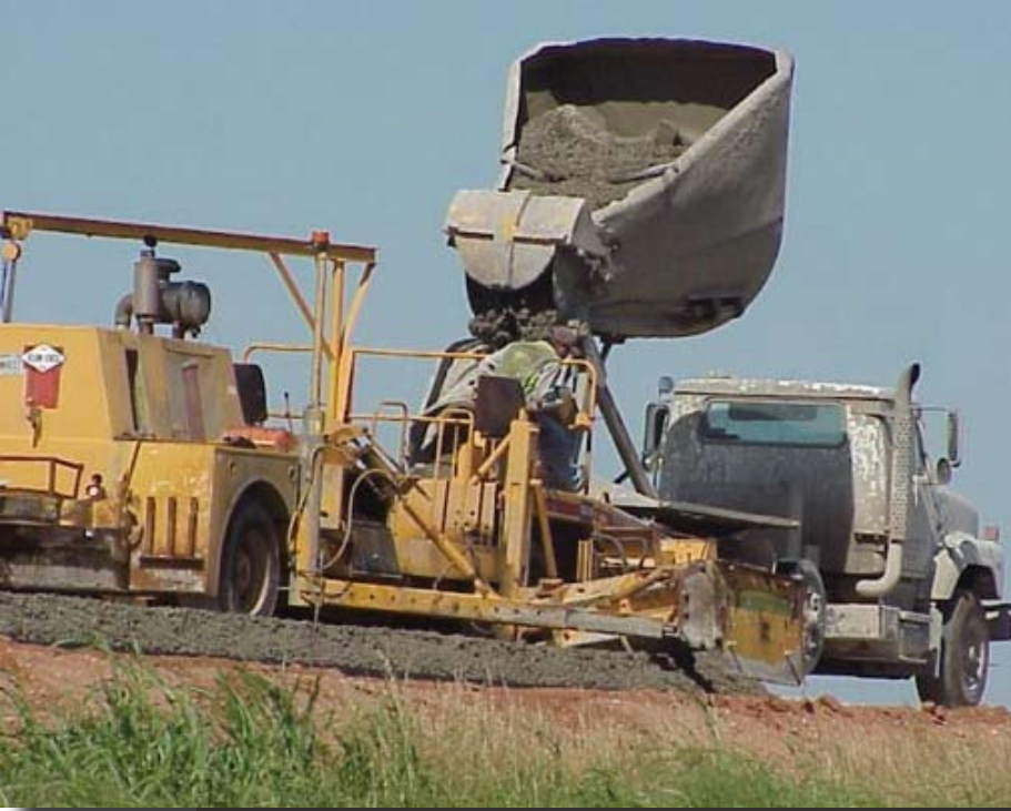
CIMARRON TURNPIKE - PAVEMENT REHABILITATION
